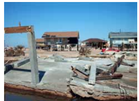
Bolivar destruction Photo by Roy Tyson/FEMA
