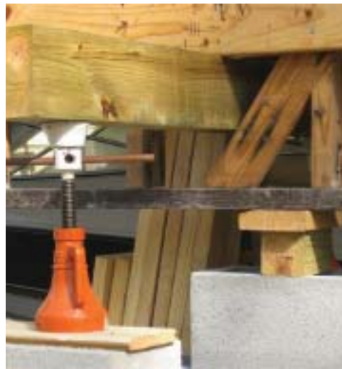
5 Ton Screw Jack used to elevate the McCloud's house.
