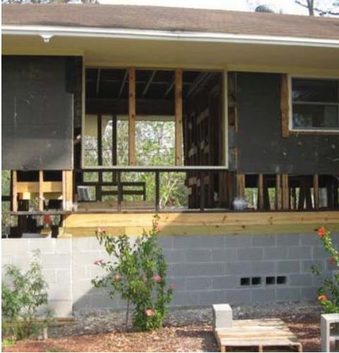
Cement block chain-wall used for elevation.
