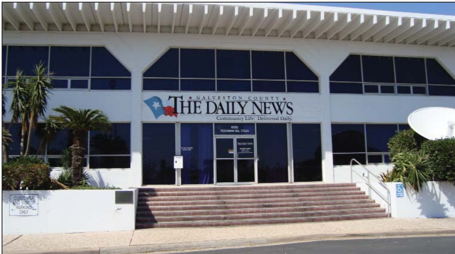
Its sturdy, elevated plant behind the seawall protected the newspaper during Hurricane Ike, but its roof was damaged.
