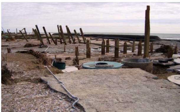
Hurricane Ike left little more than slabs and stilts on Bolivar Peninsula in Galveston County. -FEMA photo.
