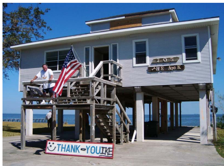
Elevating his home above the Hurricane Ike storm surge saved the house of this Galveston County home owner. -FEMA photo.
