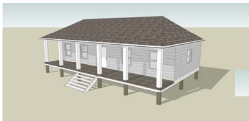
The site shows benefits of "freeboard," raising a coastal house above flood levels. – StormSmartCoasts.org
