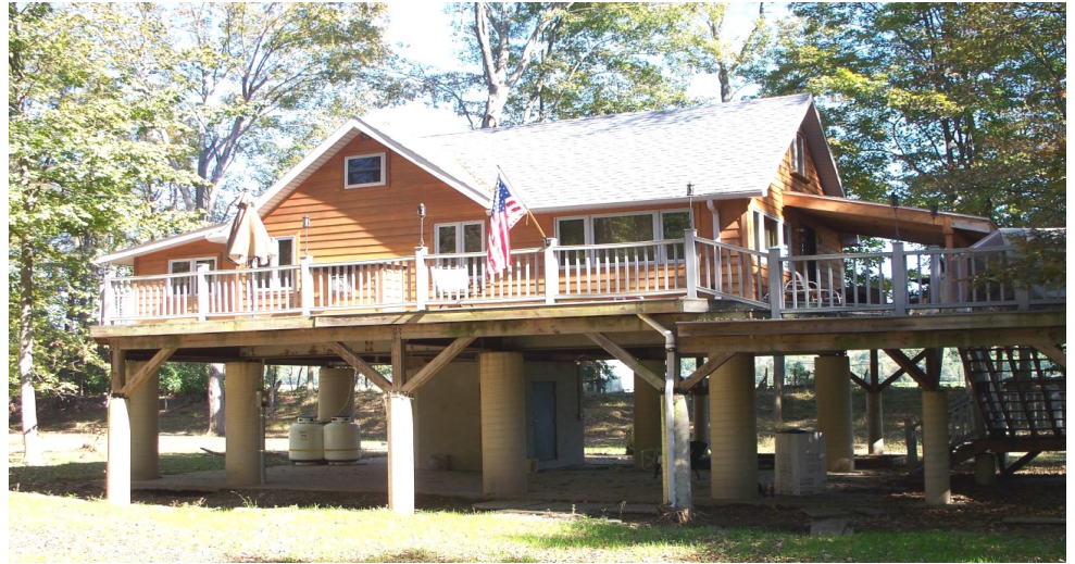
After flood damage and repair, this home was elevated on sturdy concrete piers
